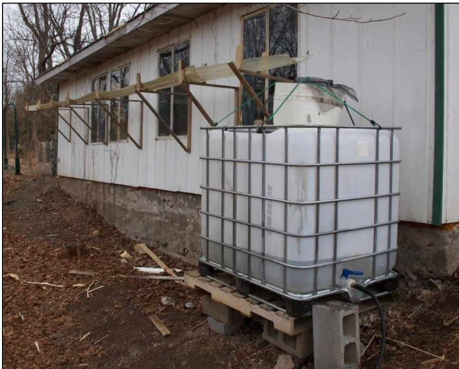
A homemade gutter made from fiberglass roofing, and a makeshift filter and first flush diverter. Notice how the gutter is several feet from the edge of the roof. This design doesn't use any pipes to collect the water.
